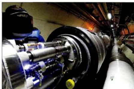
Progress on the Large Hadron Collider – welding interconnections between magnets.
